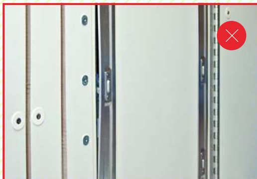
Check decompression panels and catches are in the correct position
