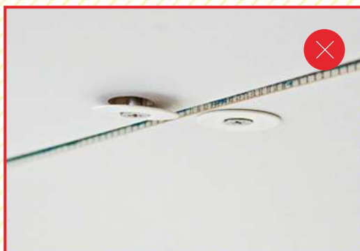
Ensure fasteners are present, tightened, and flat on the panel
