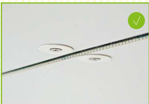
Ensure fasteners are present, tightened, and flat on the panel
