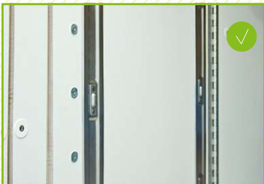
Check decompression panels and catches are in the correct position
